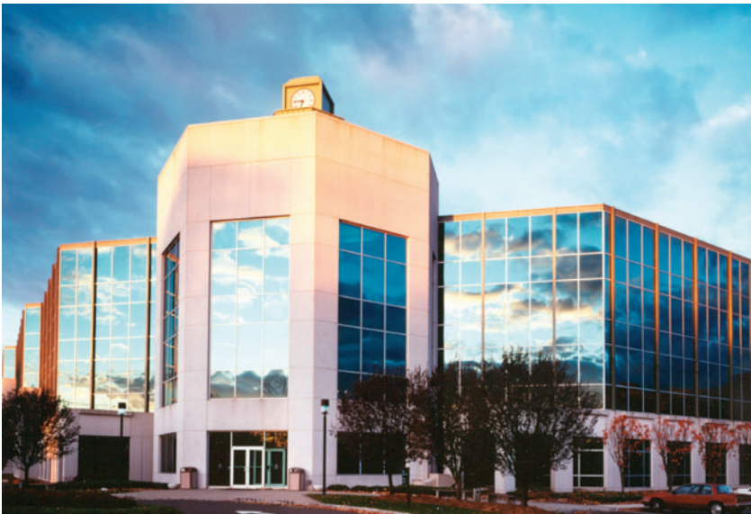
The Mack-Cali building at 20 Commerce Drive in Cranford – winner of the Energy Star Award.
